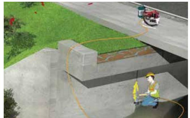
*Water leaking through cracks and joints in storm sewer pipes, culverts, manholes and other below grade structures creates a maintenance nightmare. Water carries surrounding soil into the structures resulting in erosion problems, cave-ins, potholes and broken sidewalks. Serious structural damage can occur if left untreated. You can seal the leaks and stabilize the soil inexpensively and permanently.*
